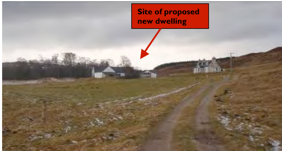
Fig. 6: Existing buildings and limited existing vegetation
